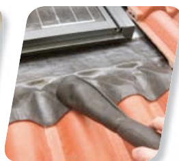
09 Install bottom flashing
