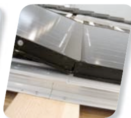
04 Install and connect photovoltaic modules
