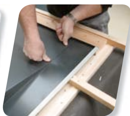
08 Install top flashing
