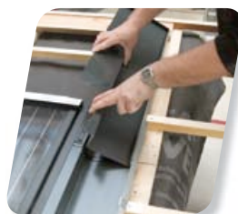
06 Install side flashing
